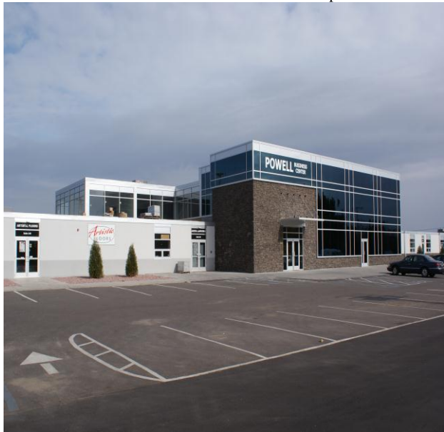
POWELL BUSINESS CENTER 7900 Excelsior Blvd Hopkins MN 55343
