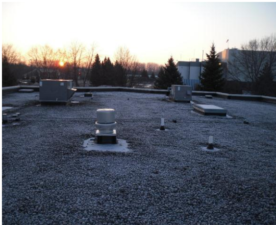
EPDM with Rock/ Ballast "Before"
