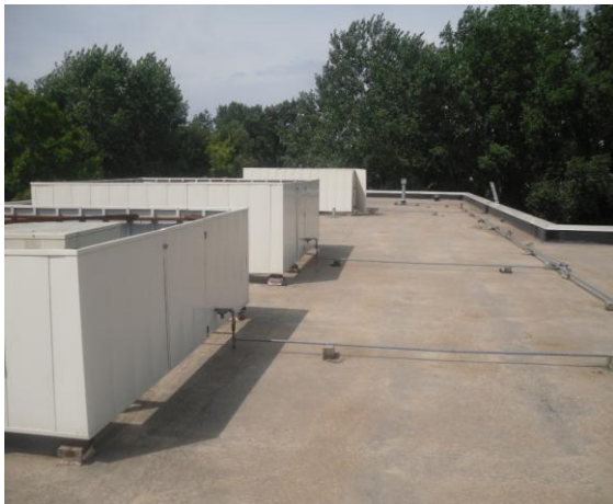
Rock/Ballast has been removed "Before"
